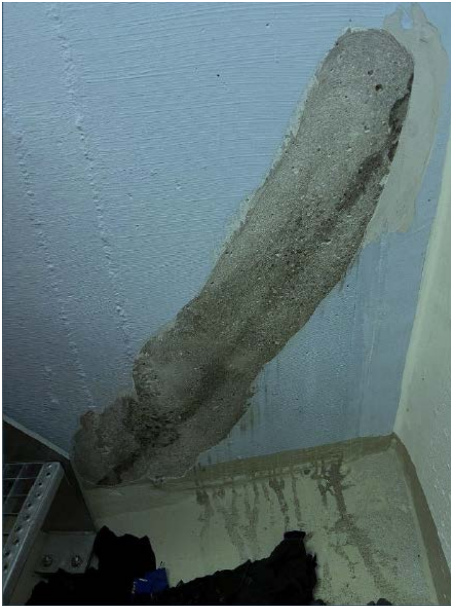
Reparatur Riss Wasserkammer "Bovel"
